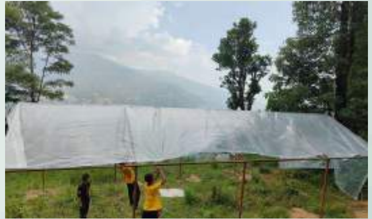
Shree Chandika Secondary School Baruwa
